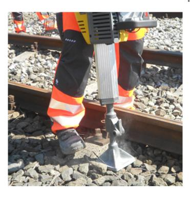
Practical ramming shoe For the compaction of railroad ballast on the edge of the rail.
