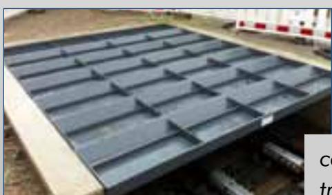
cover plates on tracks behind buffer stop in passenger railway station
